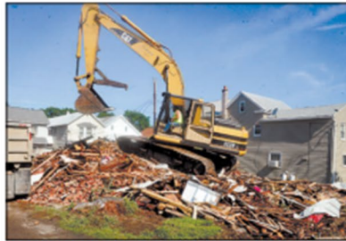
DEMOLITION WASTE is loaded into a trailer to be hauled away from the work site in Lightstreet on Tuesday morning. PHOTOS BY BILL HUGHES
