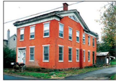
THE EARLY 19TH-CENTURY BRICK HOUSE at 1601 Main St., Lightstreet, is seen in a 2012 file photo. The blighted property was deemed unsafe and demolished Tuesday.
