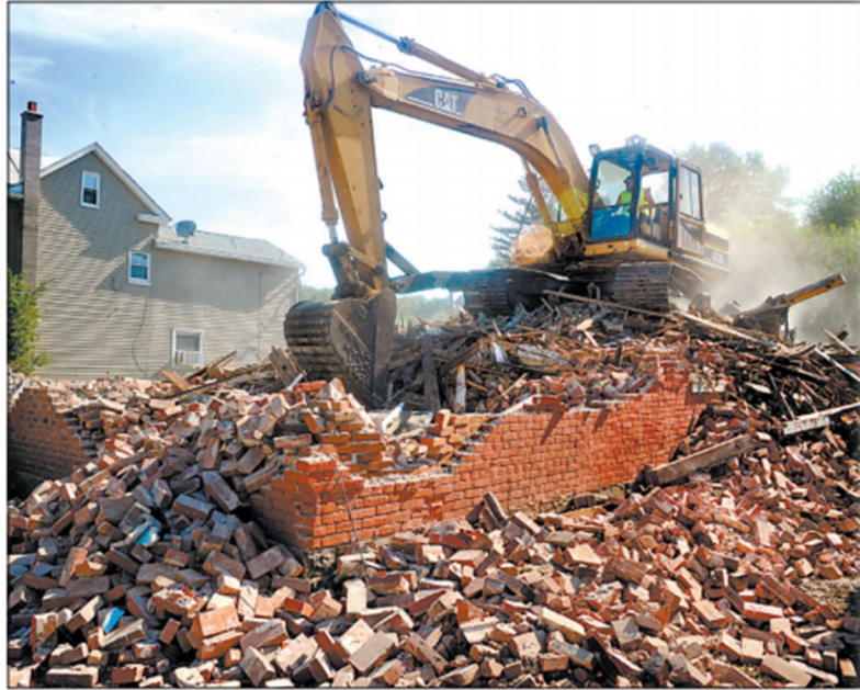
ROD FOX uses an excavator to demolish the old brick house at 1601 Main St., Lightstreet, on Tuesday morning. Fox is an equipment operator for G&M Crawford.
